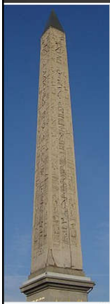
One of the two Luxor obelisks, in the Place de la Concorde in Paris: a red granite monolithic column, 23 metres (75 feet) high, including the base, which weighs over 250 metric tons (280 short tons).
